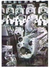
Careful inspection of main bearing housings bores, being carried out at Barton Hall Works, prior to the fitting of bearing shells
